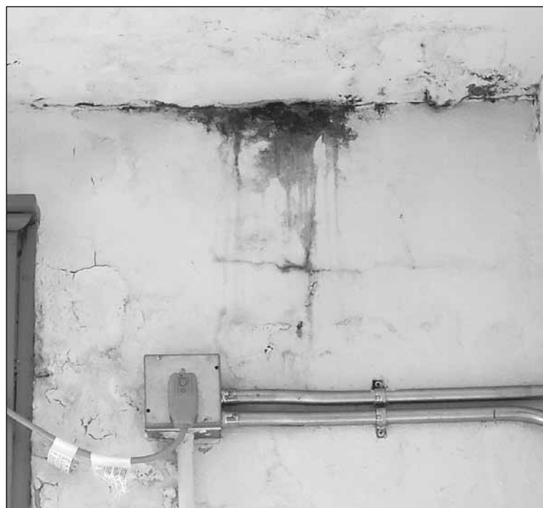
Mold on the ceiling and walls at BCC's Nichols Hall
